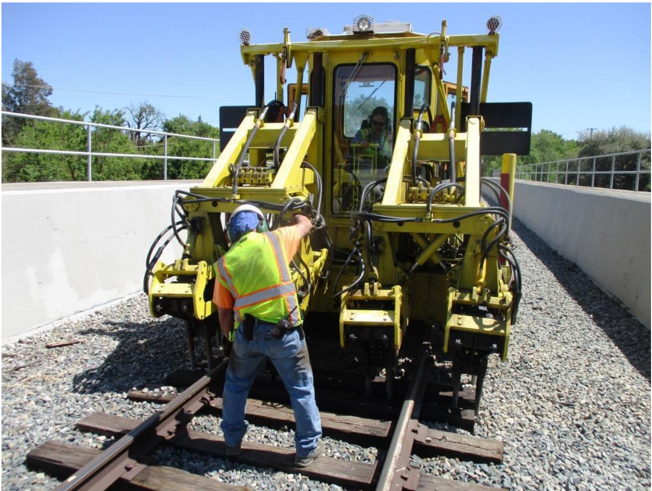
Joe acts as guide as Heather used the tamper's work-heads to position the ties properly before tamping them up
