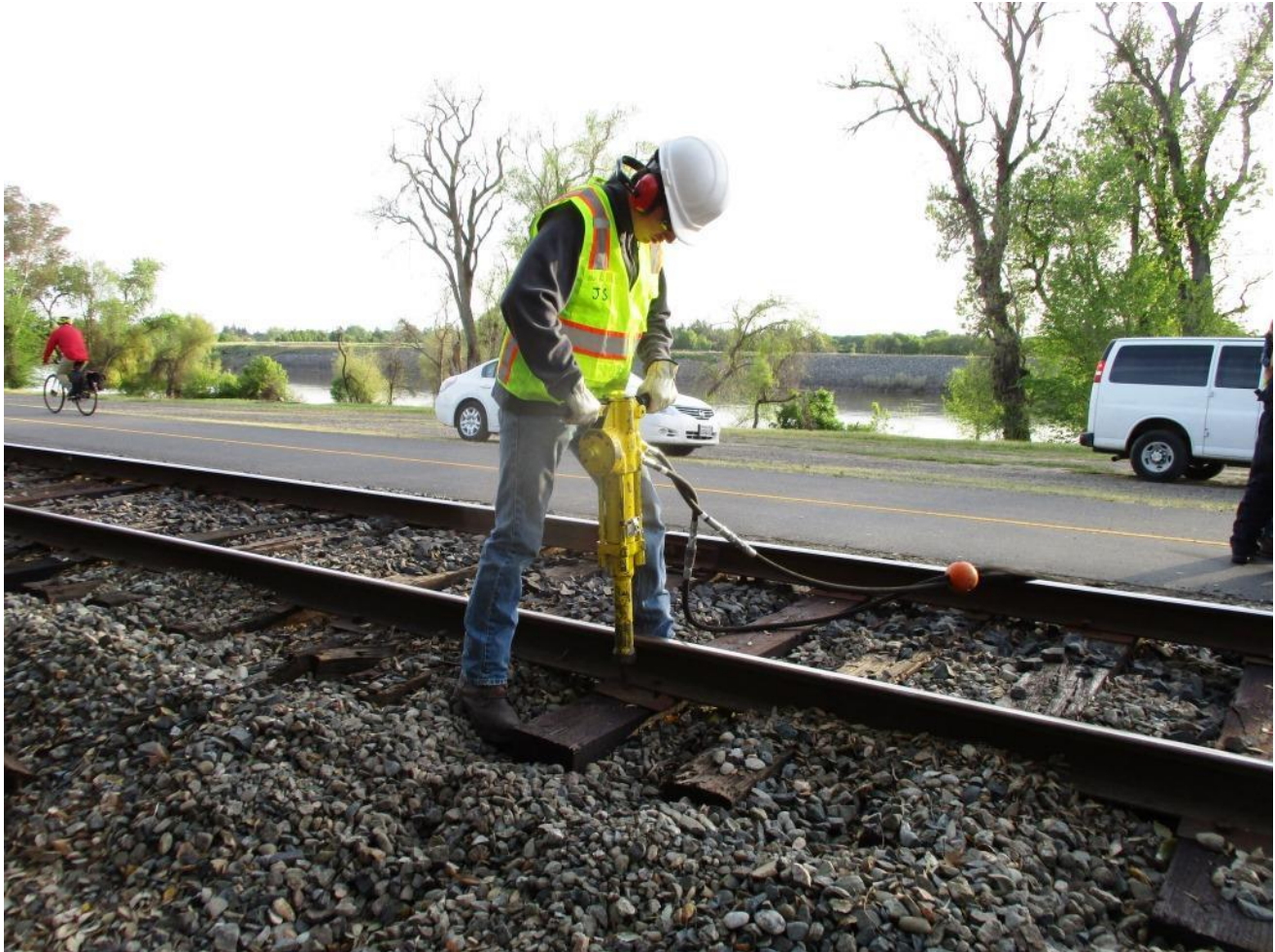
Jack's had enough of the old fashioned stuff and, instead, deploys the hydraulic spike-driver
