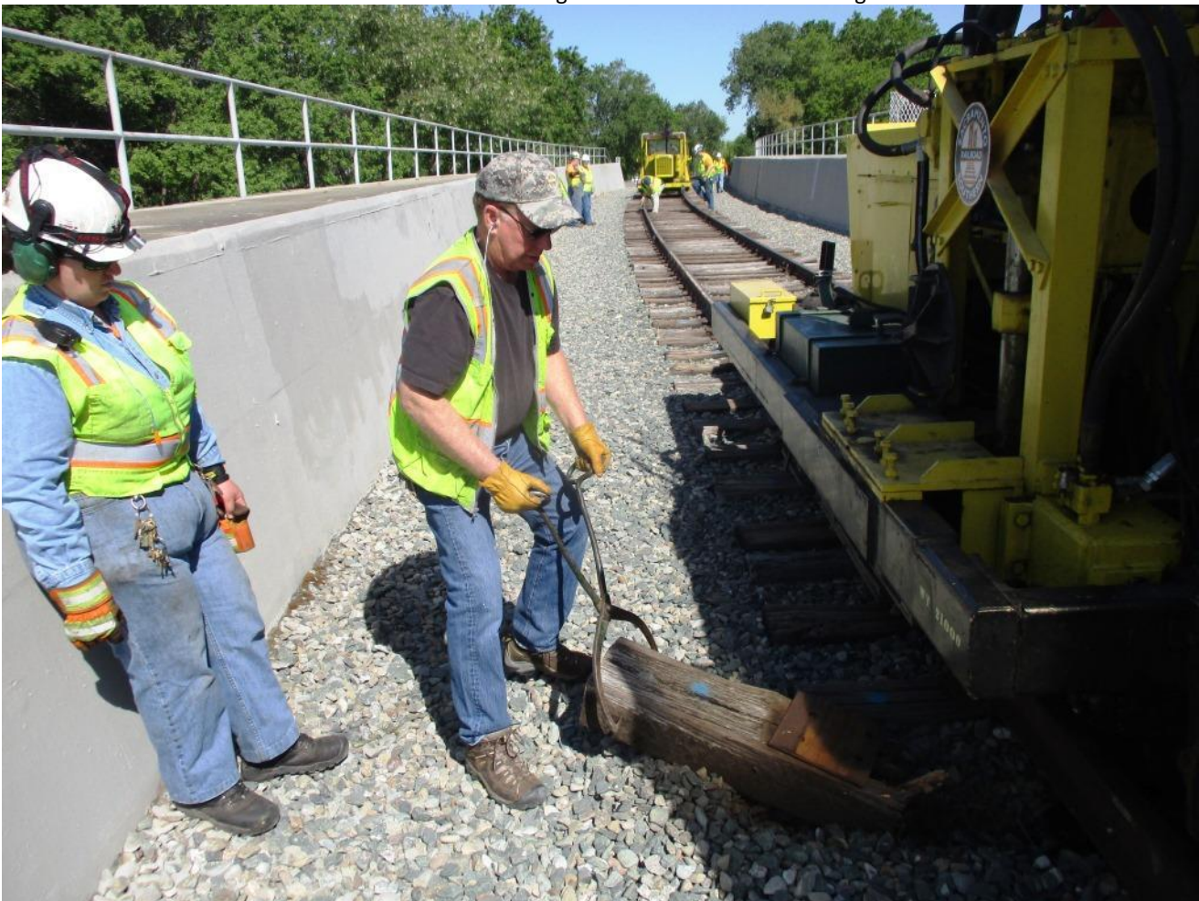
Ed M. grabs the sliced tie-debris away from the track
