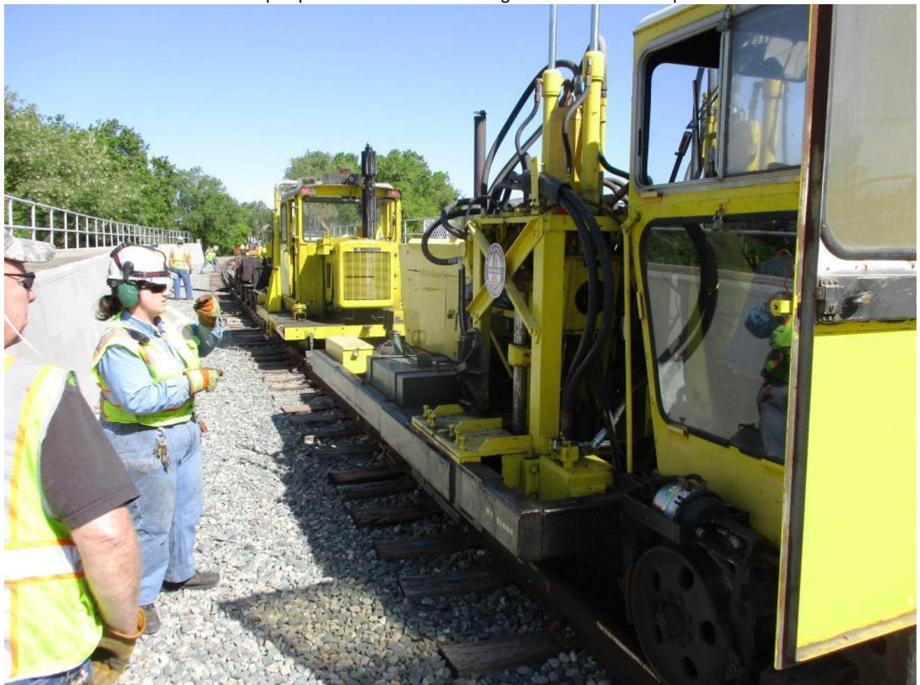
As visibility is terrible from the cab, Heather guide Frank, who is running the tie-shear, into position over the first tie to be cut
