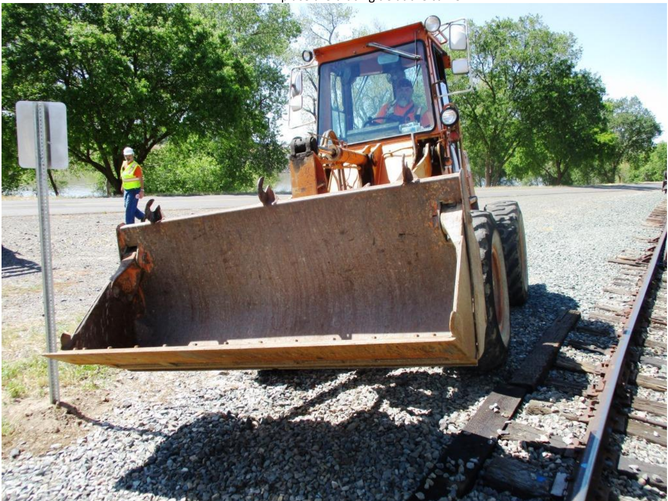
Mike F. uses the loader to compact the rock behind the bracing ties
