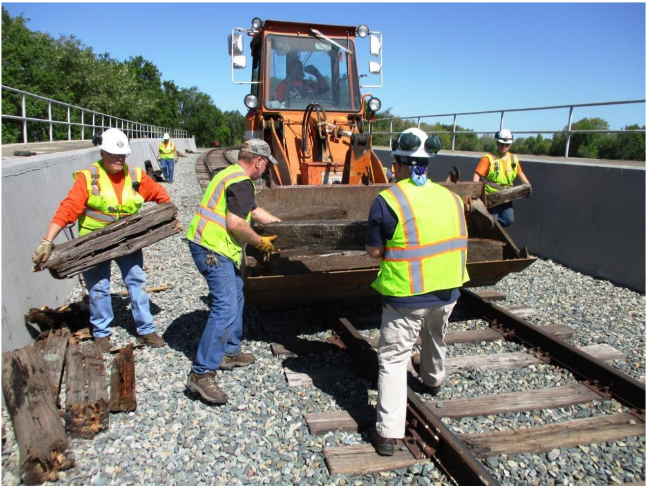
Mike F. straddles the track with the front end loader for Bill, Ed M., DJ, and Chris to load tie-debris into its bucket for disposal
