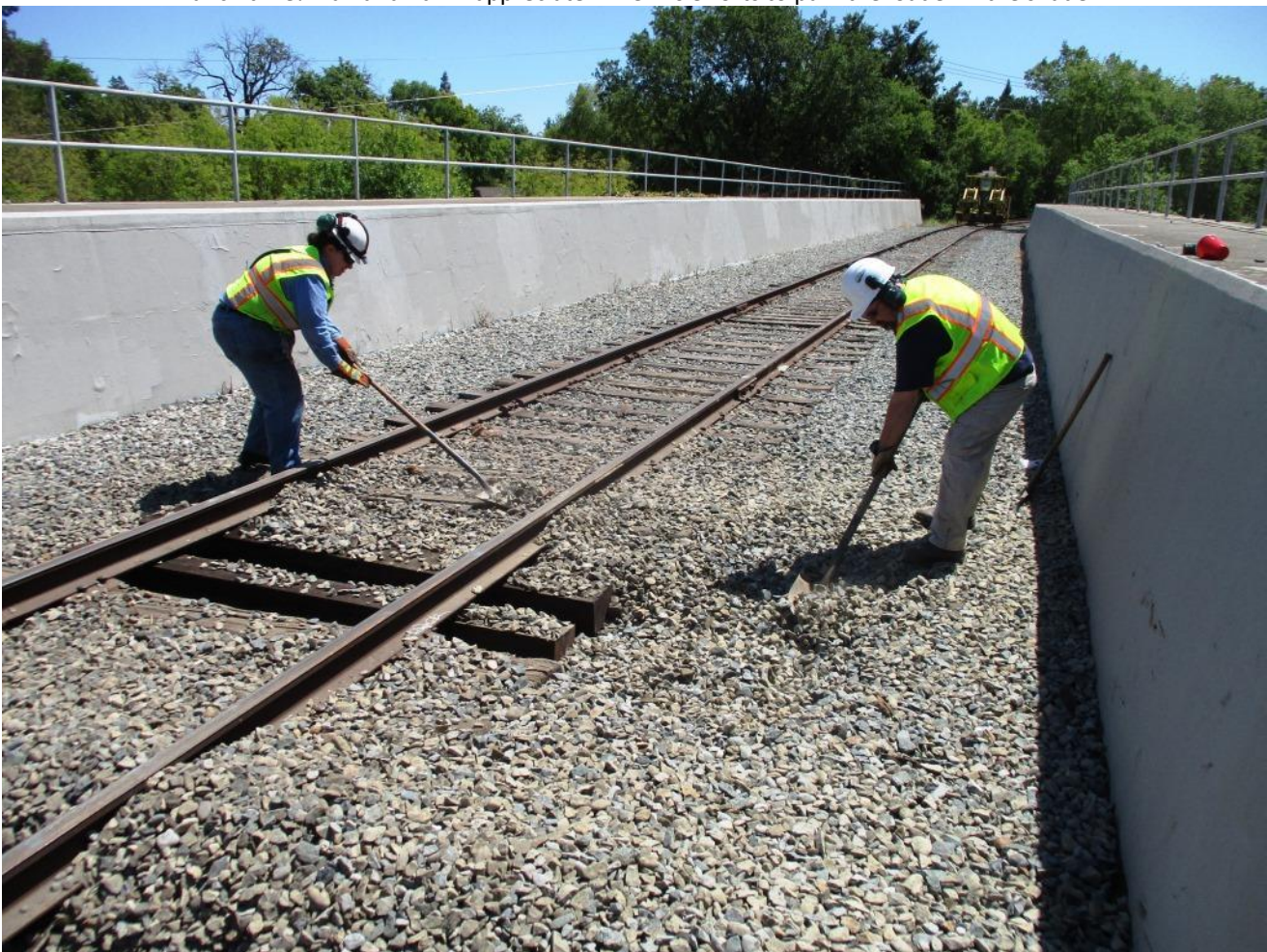
Heather and DJ shovel rock back between the ties
