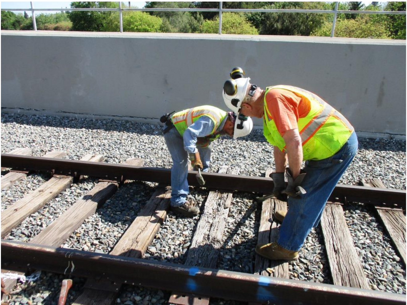
Clem nips-up the rail as Joe uses a sledge to thwack-out a tie-plate
