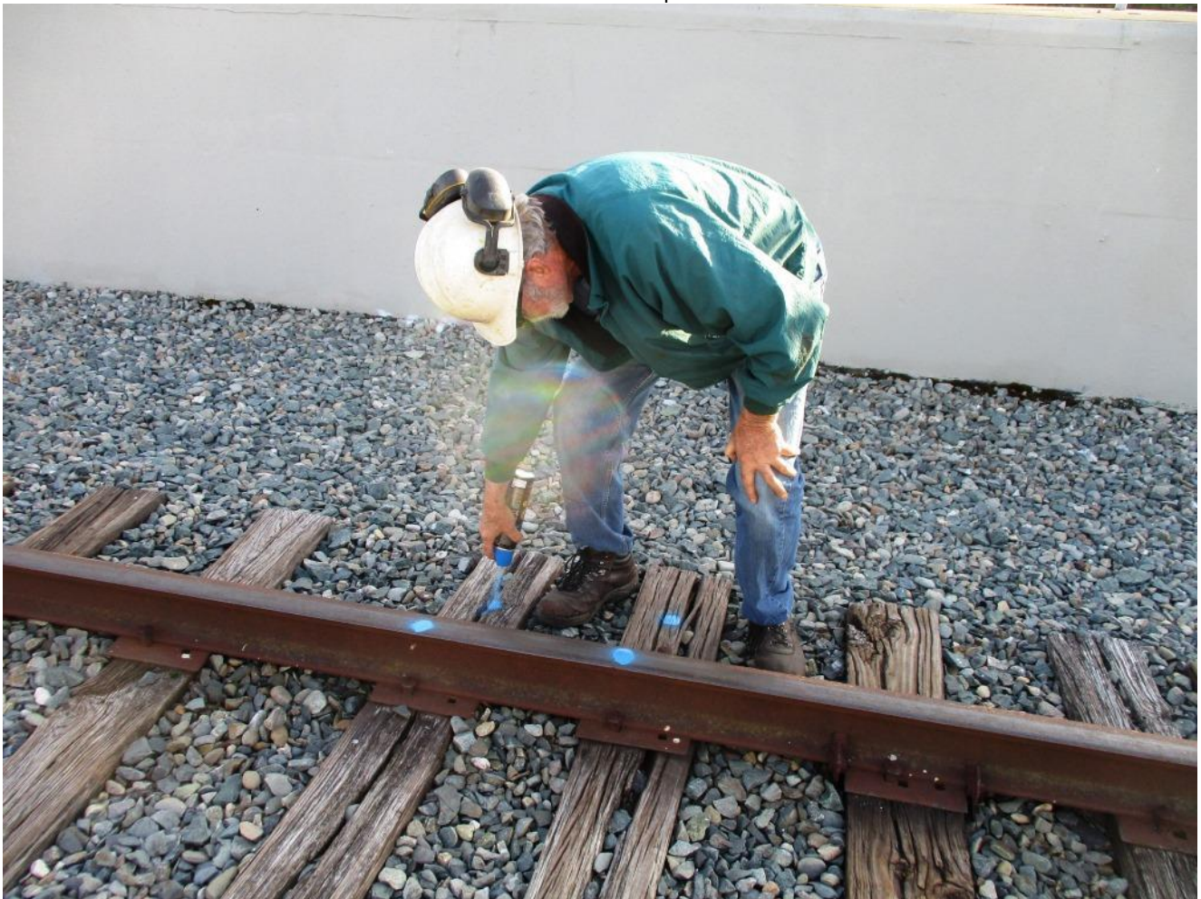
Alan marks ties to be sliced and diced on the bridge
