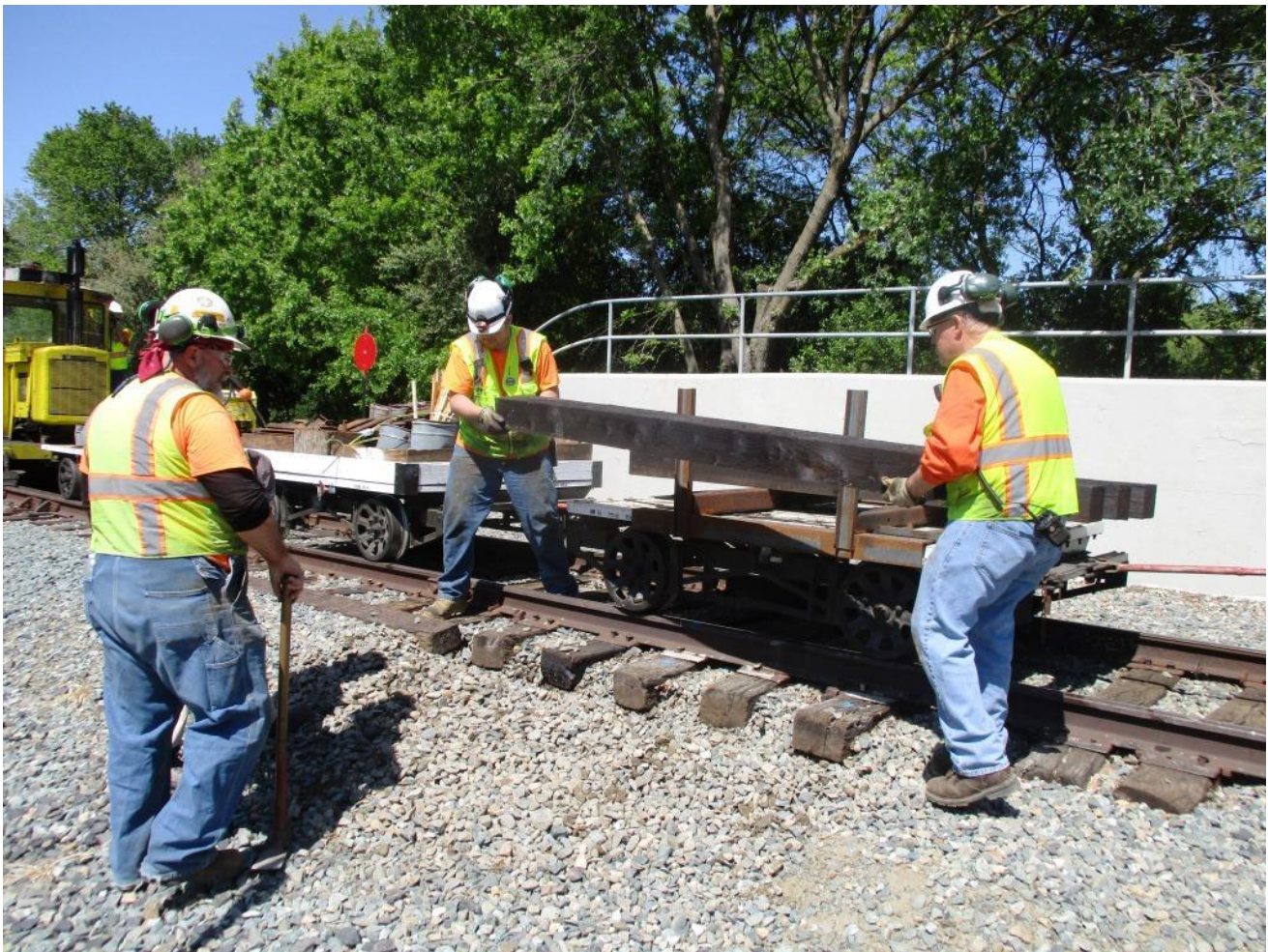
Chris and Bill place the bracing tie at the curve
