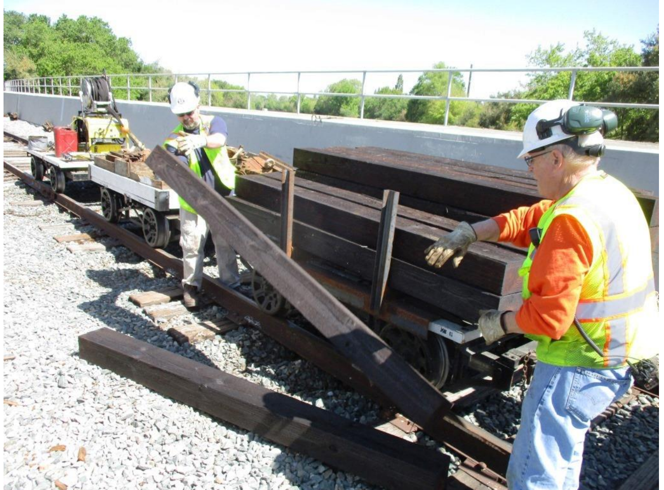
DJ and Bill deploy new ties for insertion
