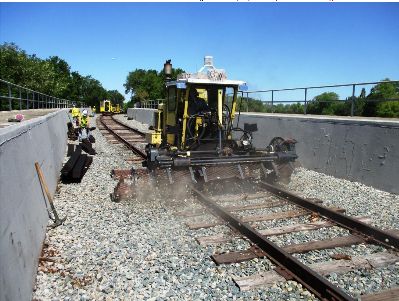
Alan, in the scarifier, digs-out a trench in the ballast-rock
