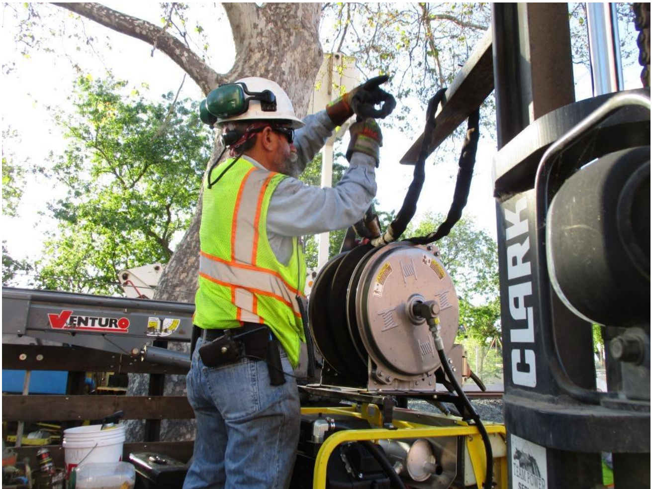
Joe straps the hydraulic power unit to the propane forklift so that it can be lifted from the truck to a flatcar
