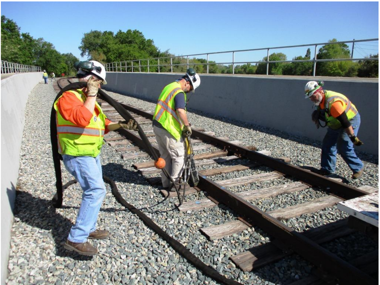
Bill handles the hydraulic hose as DJ pulls spikes on marked ties with the hydraulic spike-puller
