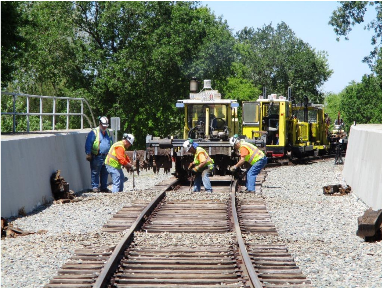
Bill, Joe, and Ed K. get the last new tie of the day inserted under the rails
