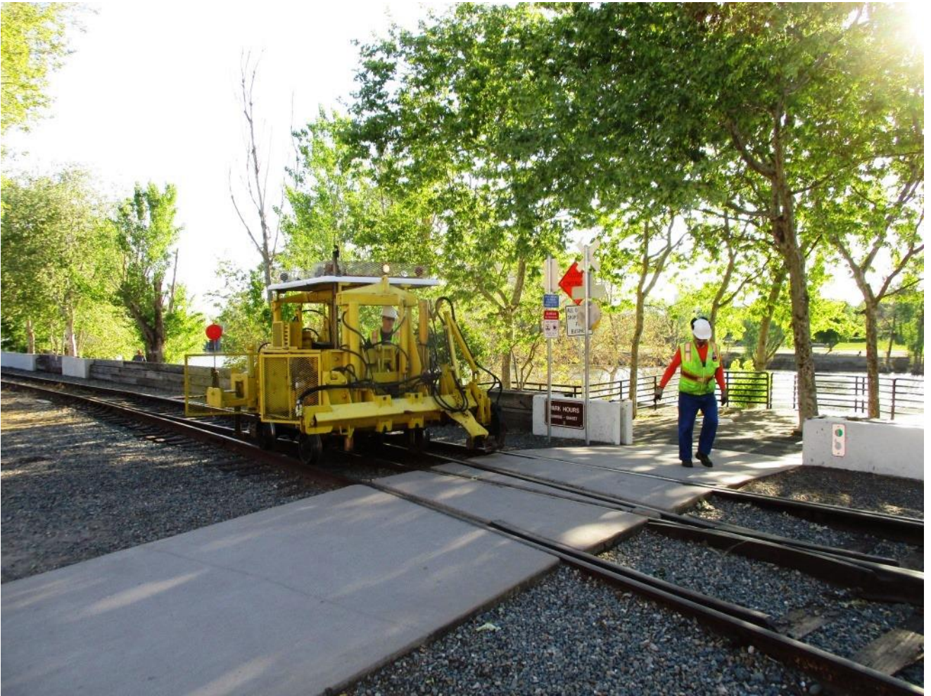
With Ed K. as brakeman, Jack moves the Jackson 125 tie-exchanger off the old 150-Track and onto the North Turntable lead
