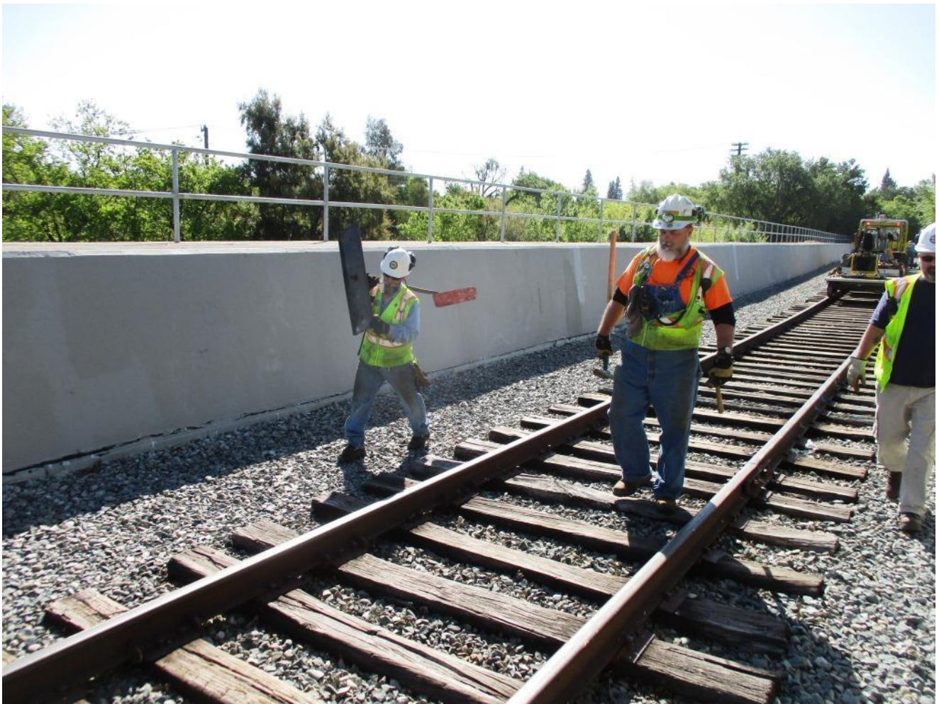
After retrieving the retractable red-flag from Sutterville Road, Joe take it to the new temporary “end of track” at MP 3.05
