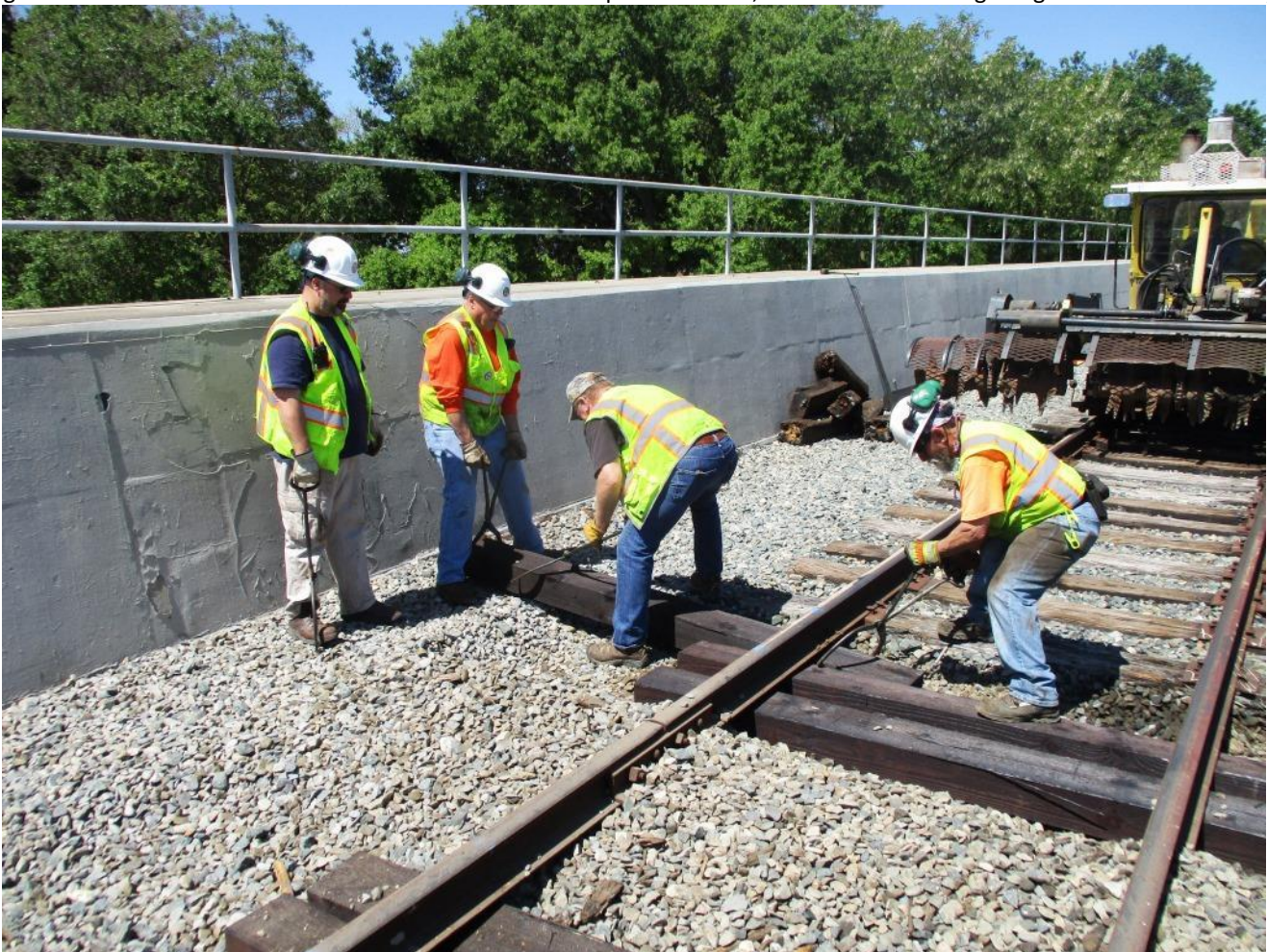
It became clear that it was easier to pull the ties in this way rather than trying to swing the grapple of the inserter to pull the ties in at an angle
