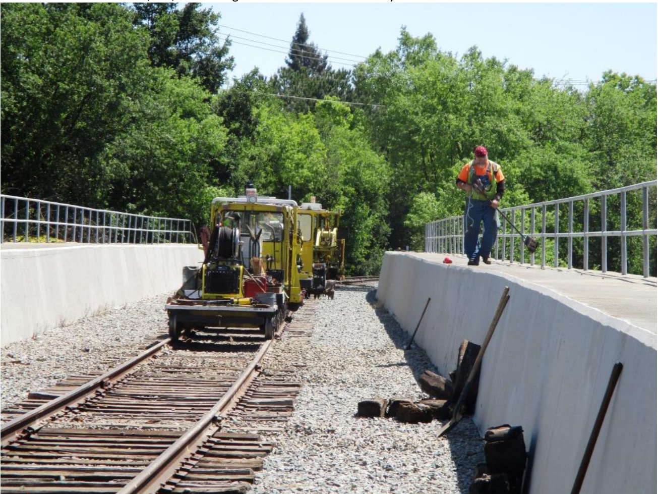
Mike F. sweeps debris off the wall of the bridge
