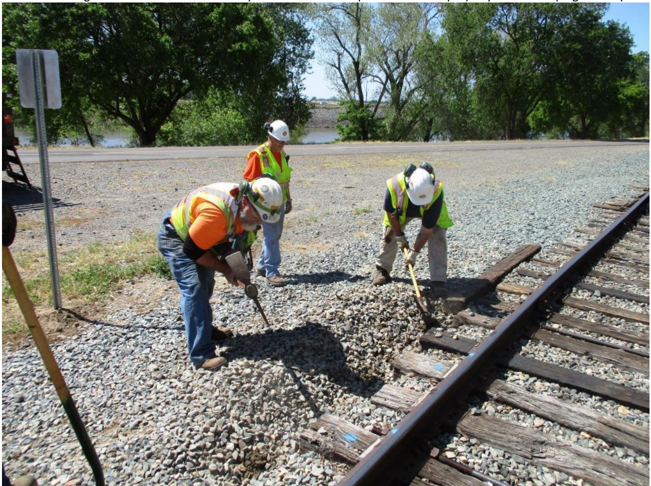
While waiting for the 3:30 train to arrive, Mike F. and DJ dig out a trench for a tie to be used as a brace in the curve south of Switch 20
